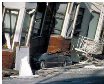
Apartment Building San Francisco, CA
